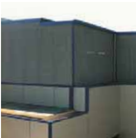
FACCIATA VENTILATA - NAPOLI - ITALIA VENTILATED CLADDING FACADE - NAPLES - ITALY
